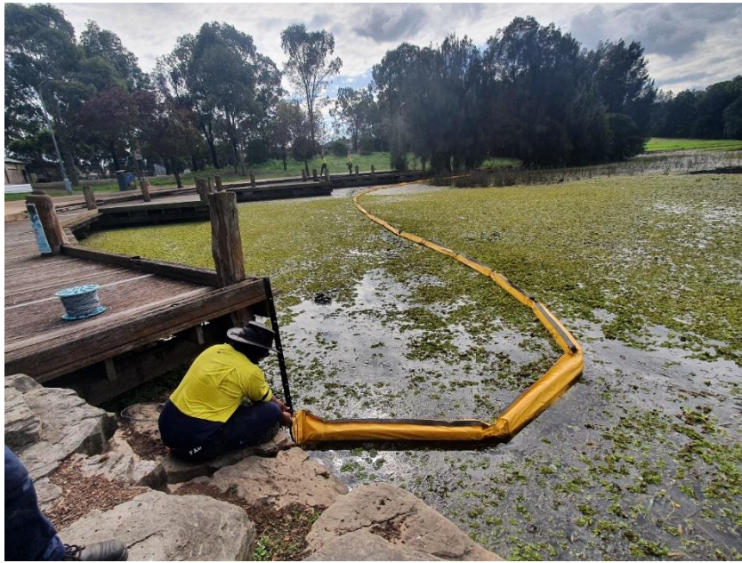
05/05/2022 Installing Aquatic weed boom at Lake Woodcroft prior to Salvinia molesta control
