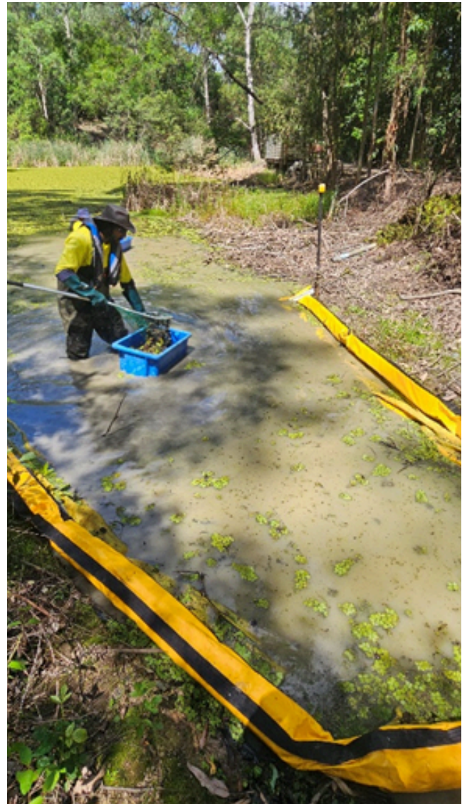
A weed boom, which acts as a floating barrier for weeds like Water Hyacinth and Salvinia.
