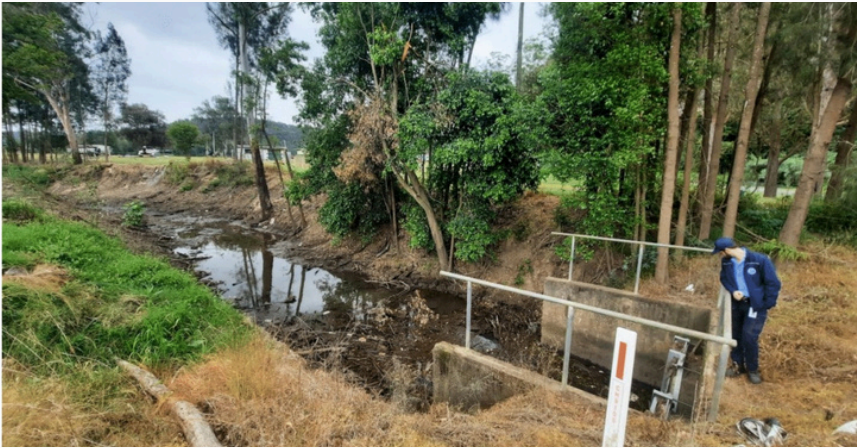
Inspecting a drainage channel for aquatic weeds.
